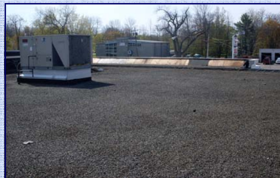
Regular, detailed inspections of roofing are crucial to asset planning.
